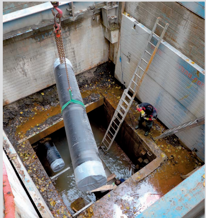
Lowering of SIMOFUSE® Pipe modules via the access structure.
