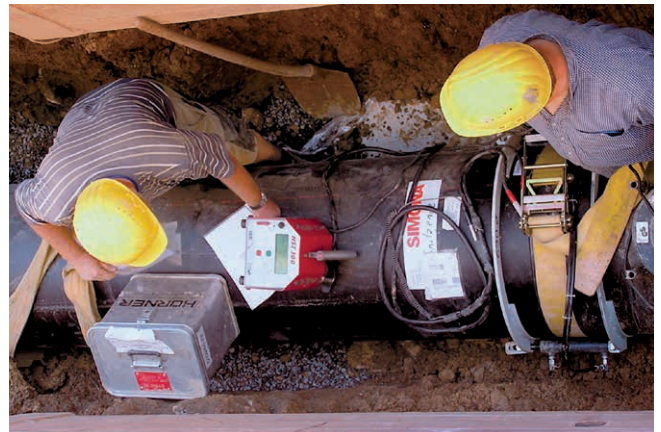
Welding is performed with a standard 40 V universal welder.
