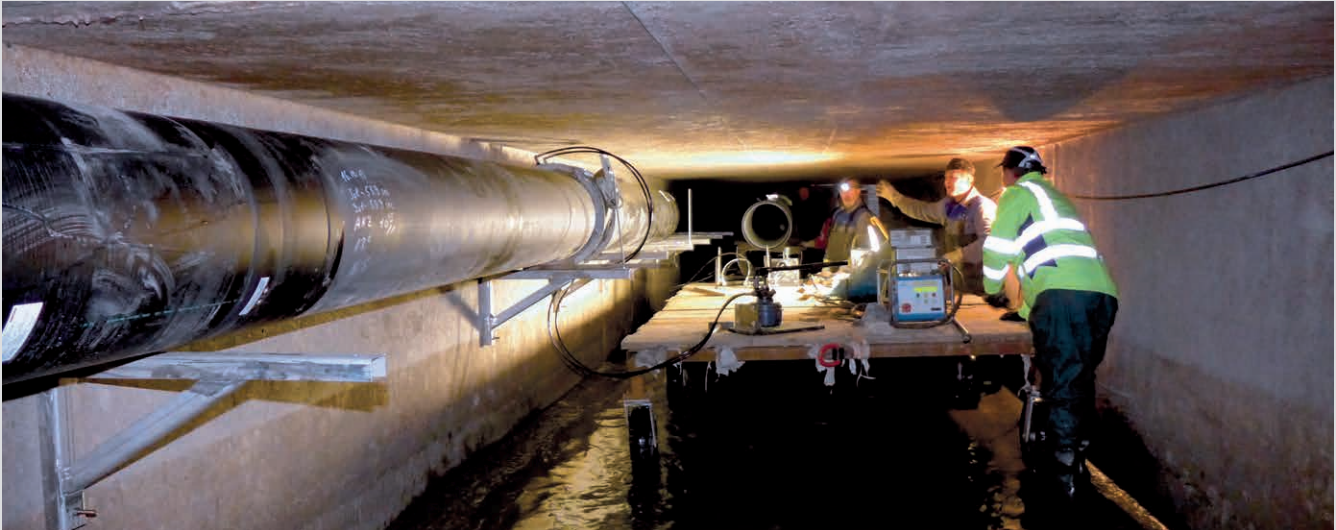
Installing the pipes in the shaft using integrated SIMOFUSE® weld connection.
