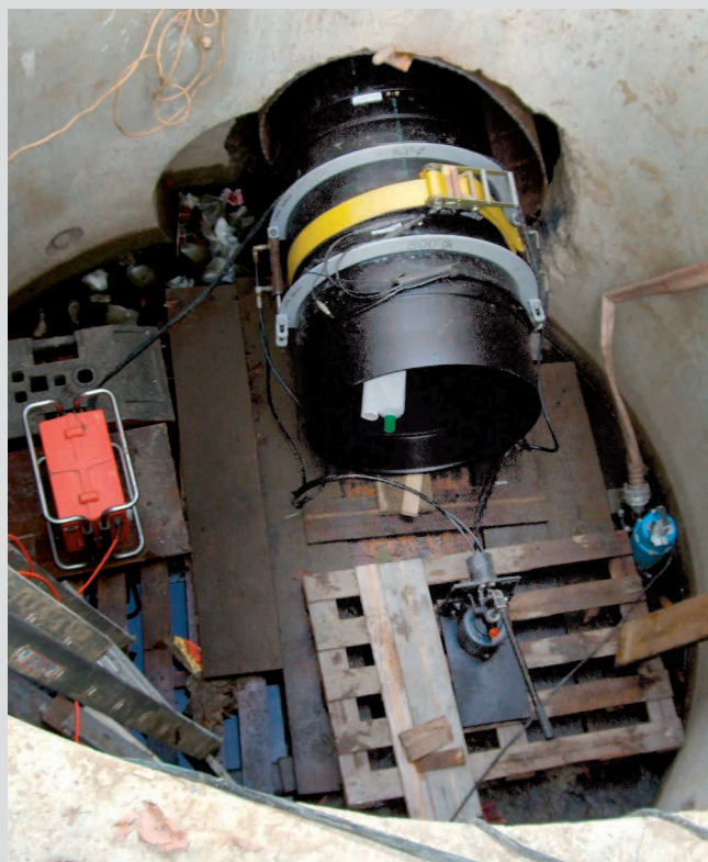
Insertion of pipe modules via the shaft.
