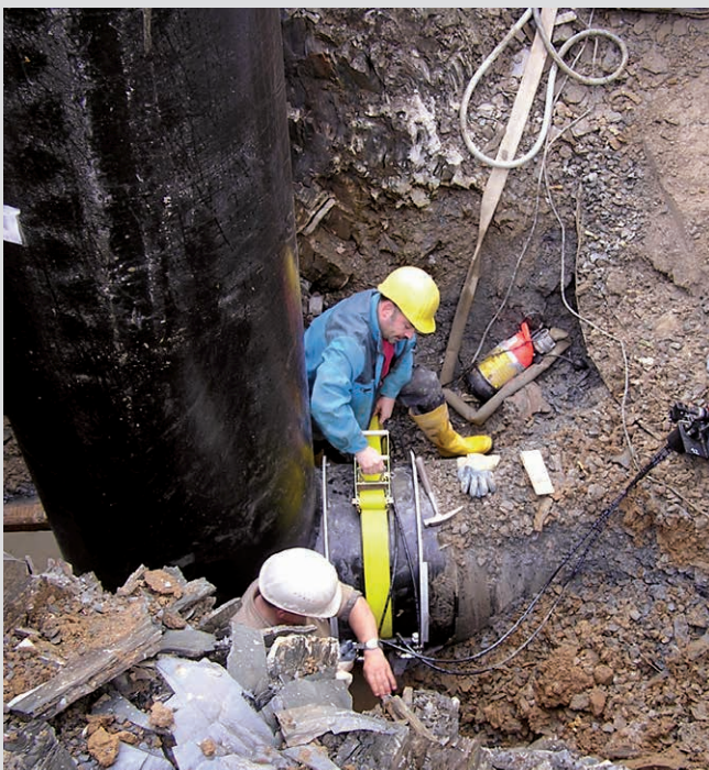
Shaft assembly at Kyrbachtal sewage treatment plant by means of SIMOFUSE® integral electrofusion connection
