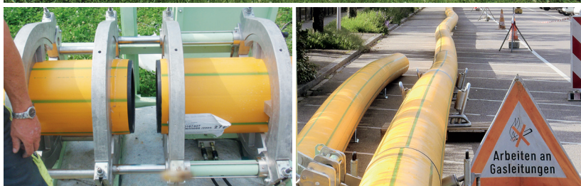
Top: delivery of the SIMONA® SPC RC-Line Pressure Pipes, section length 20 m; bottom left: butt welding of protective-jacket pipes; bottom right: pre-welded train of pipes ready for pipe insertion
